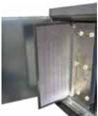
Aerosol panel filters x > 100\mu\text{m}
