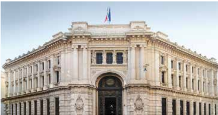
Bank of Italy Head Office, Rome (2003) - 300 fan coil units
