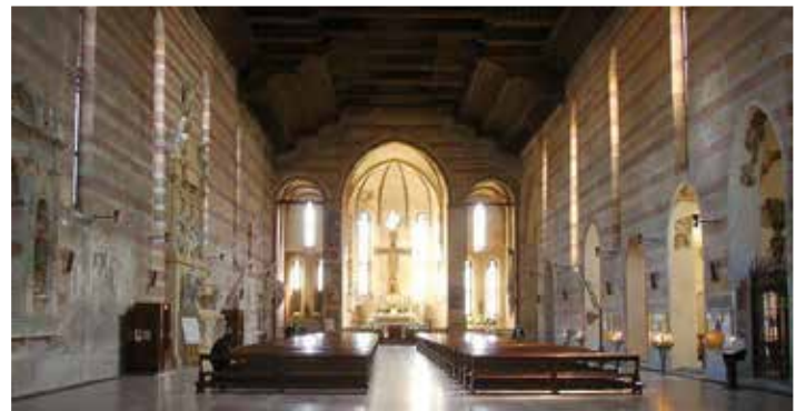
Church of the Eremitani, Padova (2011) - 40 fan coil units
