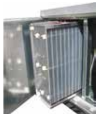
Electrostatic filters 0,01\mu\text{m} > x > 10\mu\text{m}
