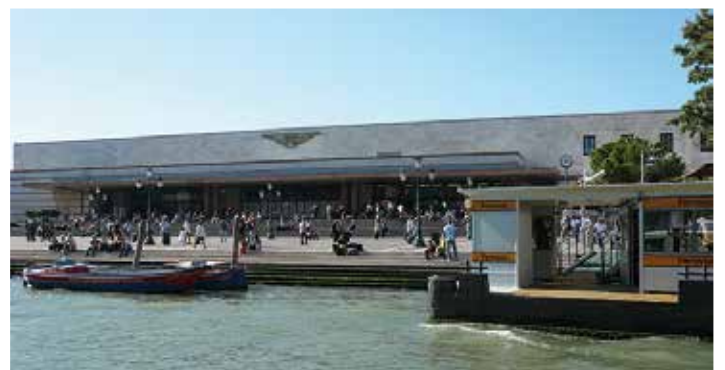
Railway Station Santa Lucia, Venice (2000) - 90 fan coil units
