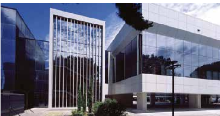
Ministry of Mercantile Marine, Rome (1998) - 200 fan coil units
